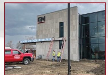
New location mid construction
